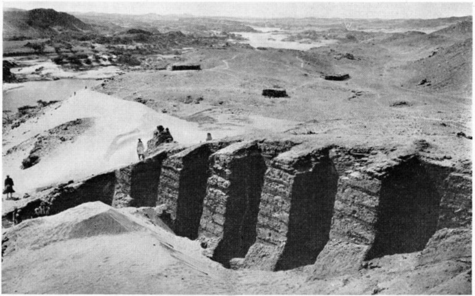
Fig. 7. Uronarti Fort; outside of massive wall; looking south, with Semna East (marked E) and Semna West (marked W) in the distance; note the horizontal wooden beams strengthening the face of the wall. December 20, 1928.
